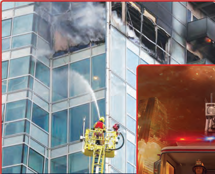
DIFFICULTY REACHING HIGHER FLOORS OF THE BUILDING
